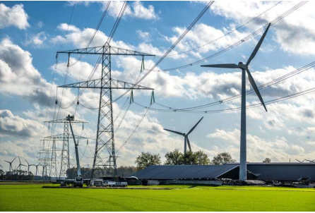
Green electricity generation and high voltage network
